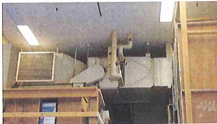
Figure M8: Heating Ventilating Unit
