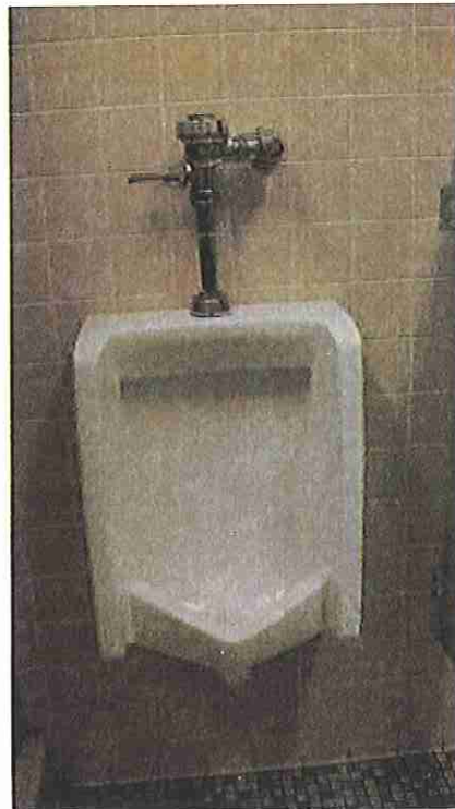
Figure P4: Urinal with flush valve
