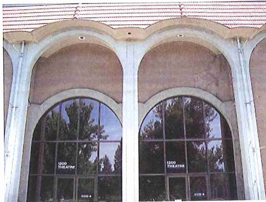
Figure 6 – Typical Exterior Perimeter Lighting
