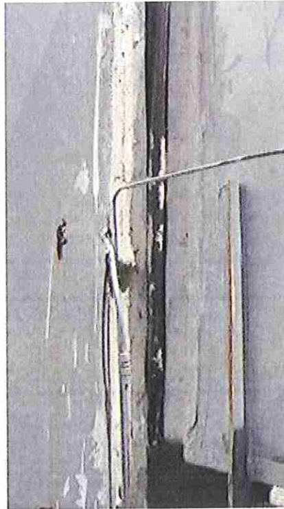
Figure M4: AHU's flex connector
